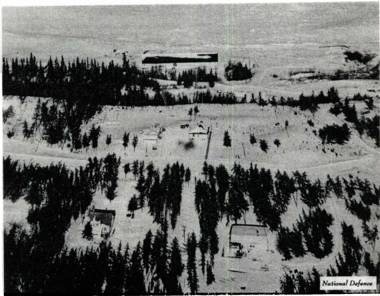
The present modern station (centre, above) is up-to-date in every respect, as are the married quarters (lower left) and single men's quarters (lower right)
